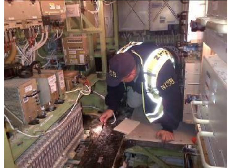
Electrical equipment bay – Boston event
